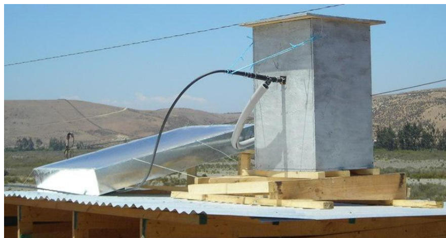
Image 2: Solar water heater built and installed at the locality of Mincha Norte (Coquimbo Region)
