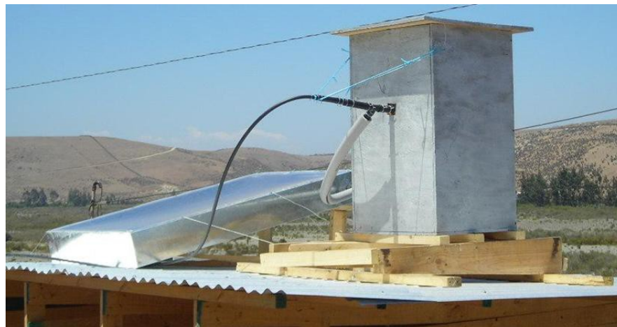
Image 2: Solar water heater built and installed at the locality of Mincha Norte (Coquimbo Region)
