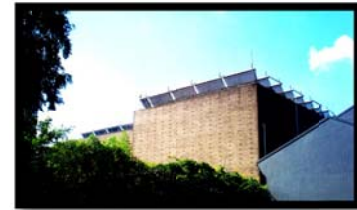
Fig1. Solar Energy Collectors
